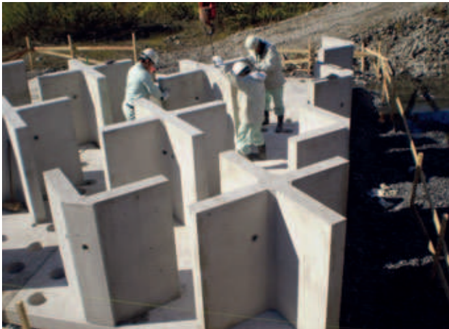
Figures 5 and 6: Assembly of the X-shaped Stormwater Reservoir
